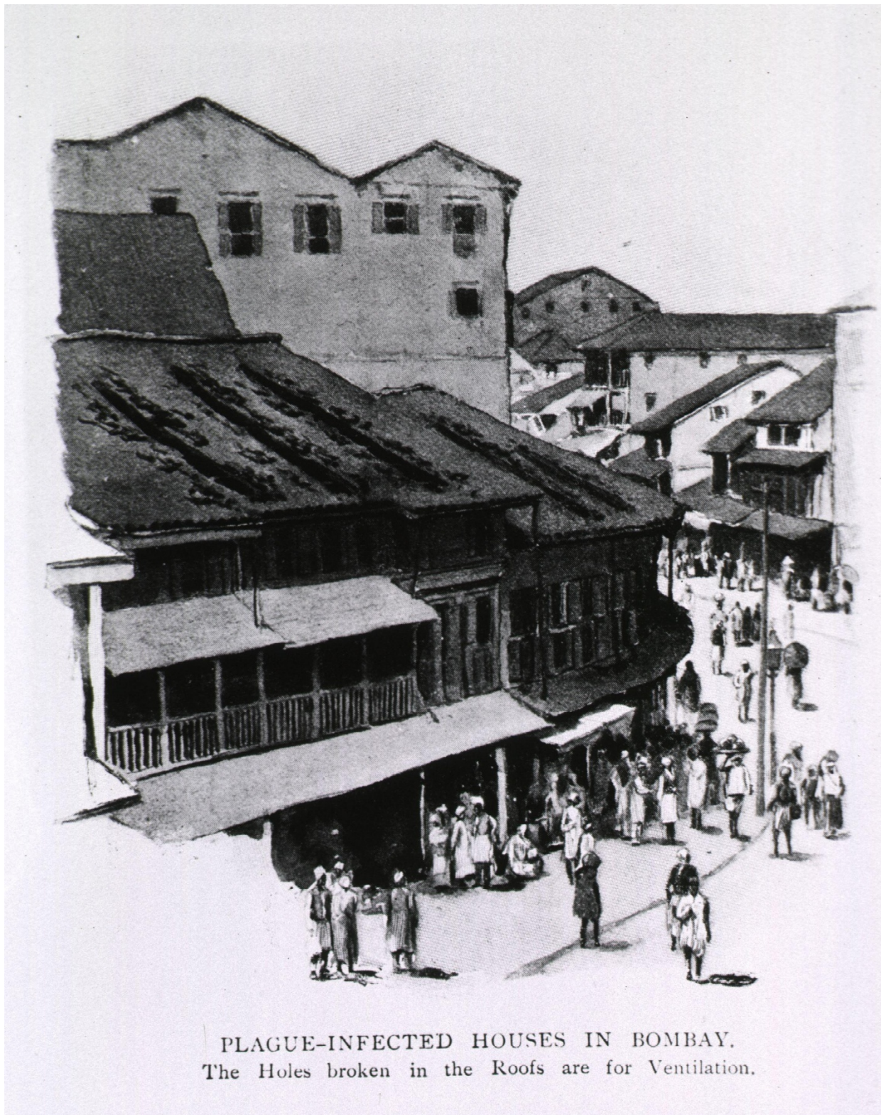
Fig. 10. Holes carved on the roof of Plague Infected Houses, Bombay. 210
